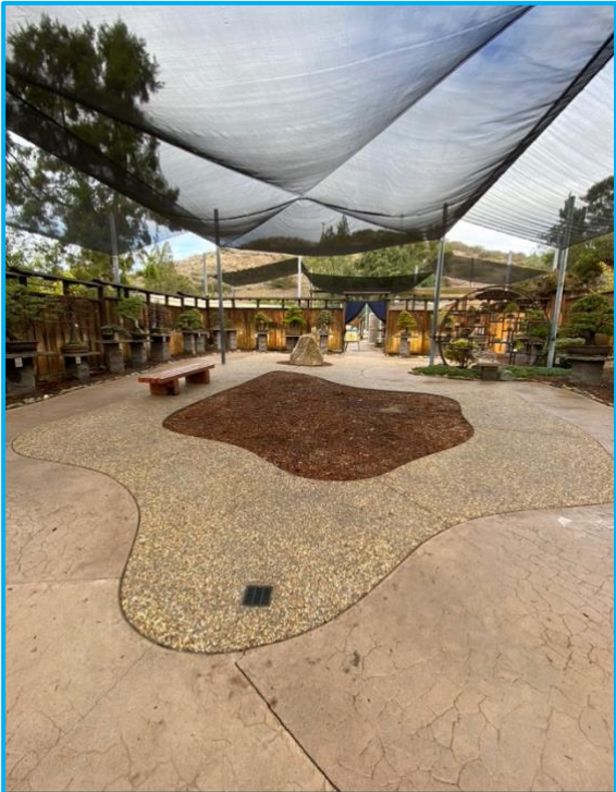
New hardscape in upper level of Pavilion
