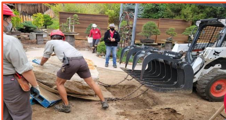
Installing the Rock
