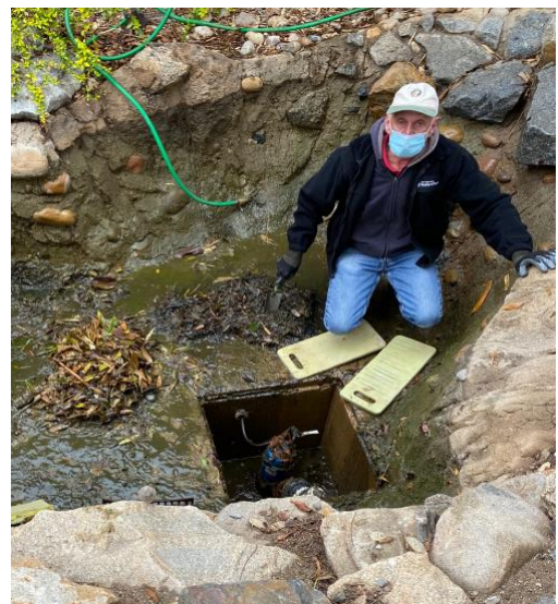
Mark Edgar cleaning lower pond drainage trap
