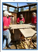
Using our hydraulic lift carts, we manage to minimize lifting this top with muscle power. We used the lift cart to set the top on the 38" high pedestals, then we used the cart to lift each end of the stone to apply adhesive to secure the top to the pedestal blocks.
