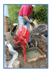
The team has developed a smooth and efficient routine for pouring the foundations and setting the blocks in place. About 260 man hours have been spent building 20 pedestal bases.
