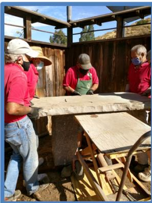
Using our hydraulic lift carts, we manage to minimize lifting this top with muscle power. We used the lift cart to set the top on the 38" high pedestals, then we used the cart to lift each end of the stone to apply adhesive to secure the top to the pedestal blocks.
