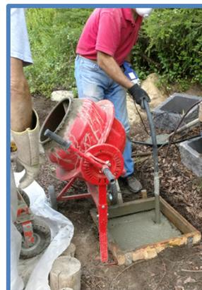
The team has developed a smooth and efficient routine for pouring the foundations and setting the blocks in place. About 260 man hours have been spent building 20 pedestal bases.
